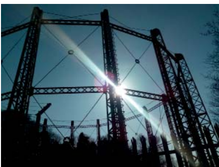
One of the gas holders before these were demolished in 2018 (Photo: Kevin Vincent)
